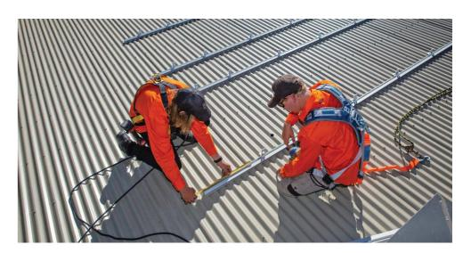
Solar panels are securely mounted onto the aluminum mounting system that's installed directly onto your roof. All our mounting systems are installed to comply with the engineering certification, panel manufacturer specifications and AS/NZS 1170.2:2011 - which includes installing additional footings for our wind region.
